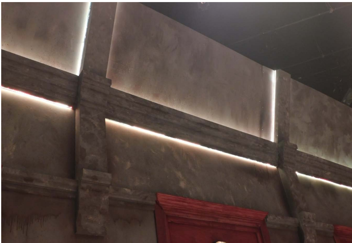
Close-Up of Set: Foam Molding and LED Tape
