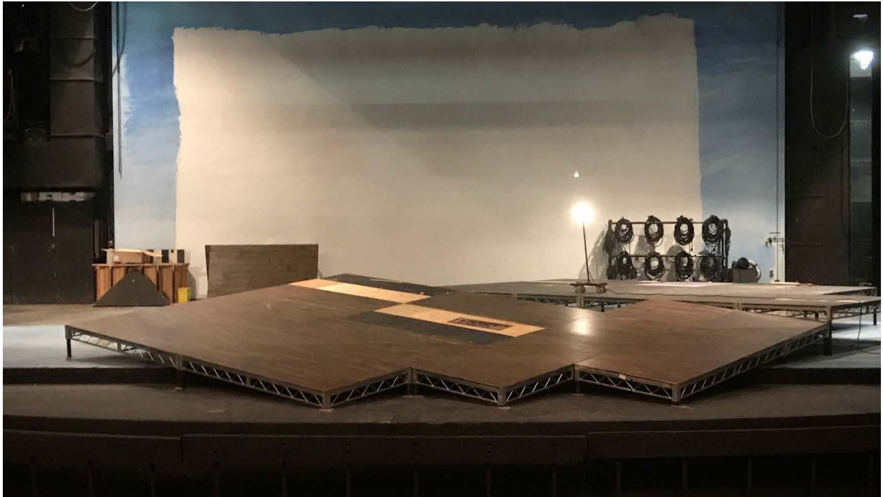
Raked Deck installed into the theater.
